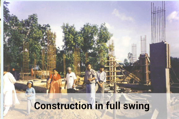
Brick by brick, pillar by pillar
